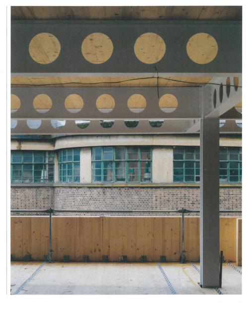
A hybrid timber and steel structure features at 6 Orsman Road, a £10m flexible workspace project beside the Regent's Canal in Hackney, east London, designed by Waugh Thistleton for Boultbee Brooks Real Estate.
